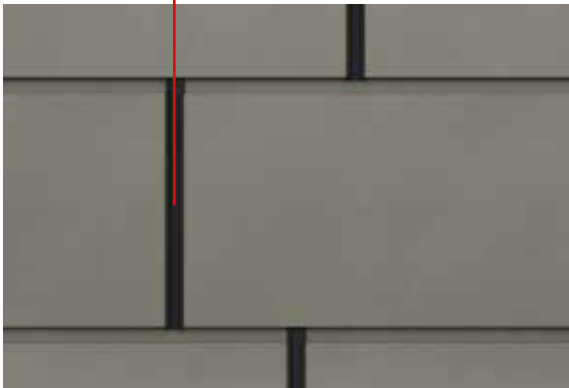
Joining using joint cover Z-301
